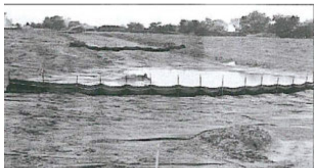
Properly installed silt fence detains water for sedimentation to occur
