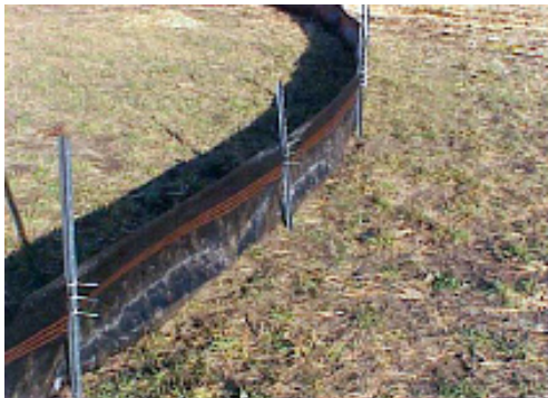
Consistent, dependable installations.
